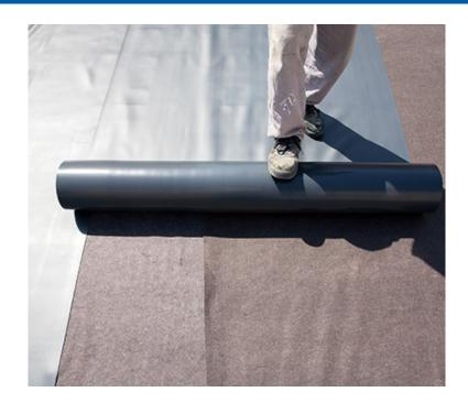
The transport business required a low-thickness waterproofing membrane, which offered protection to the bridge decks and also met the criteria defined by Milan Metropolitan office (MM). The chosen system had to offer resistance to hot asphalt, provide complete adhesion and be easy to apply.
